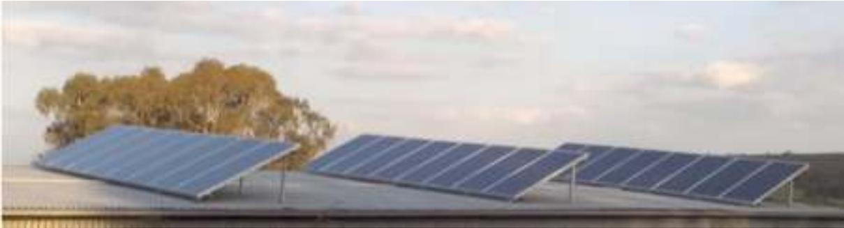
*Tilt frames allow you to set the tilt angle on a flat roof (credit: Antai Solar)*
